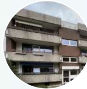
First external project, Düsseldorf
